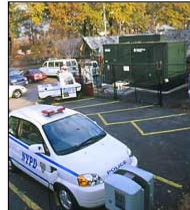
A 250-kilowatt phosphoric acid fuel cell powers a police station and electric vehicle recharging station in New York's Central Park
