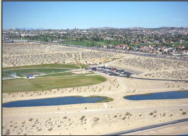
Constructed wetlands in Boulder City, Nevada
