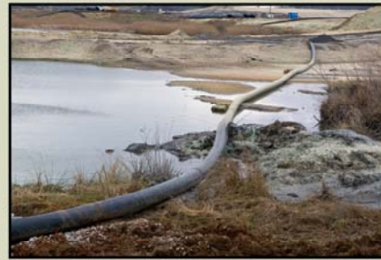
A dredging operation
