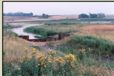
Installation of a water control structure
