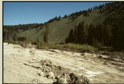
Highway construction in a wetland
